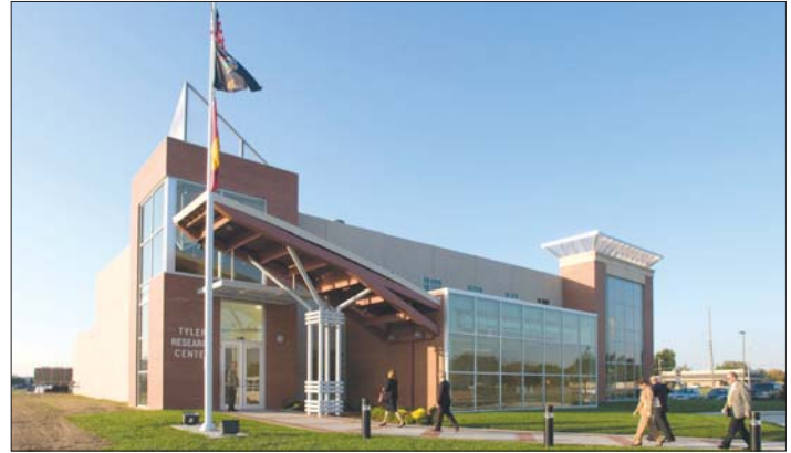
Tyler Research Center opened in September, launching state of the art bio-based products at R&D facilities for Pittsburg State University. Photo courtesy of PSU.
